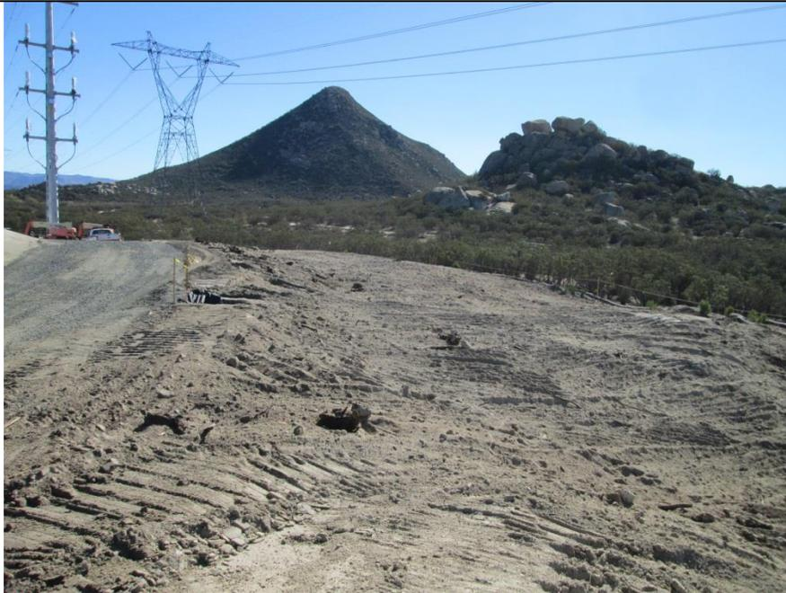
**Photo 4:** A pull site near SP-38 is decompacted and recontoured in accordance with MM-BIO-1D.
