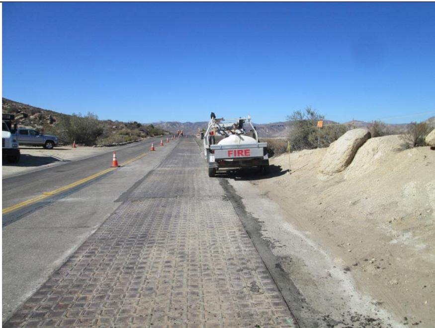
**Photo 2:** Fire equipment is maintained onsite during construction activities in accordance with MM-FF-1 and the Construction Fire Prevention Plan.
