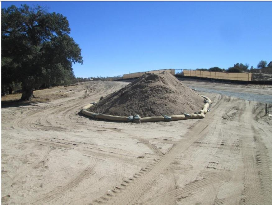
**Photo 6:** Topsoil is staged at the Boulevard Substation Rebuild site for use during restoration efforts in accordance with MM-BIO-1D.
