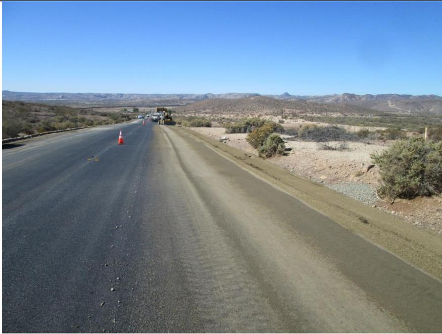
**Photo 1:** Construction crews were observed paving Old Highway 80 along the 138 kV underground alignment to repair roads damaged in accordance with MM-TRA-2.
