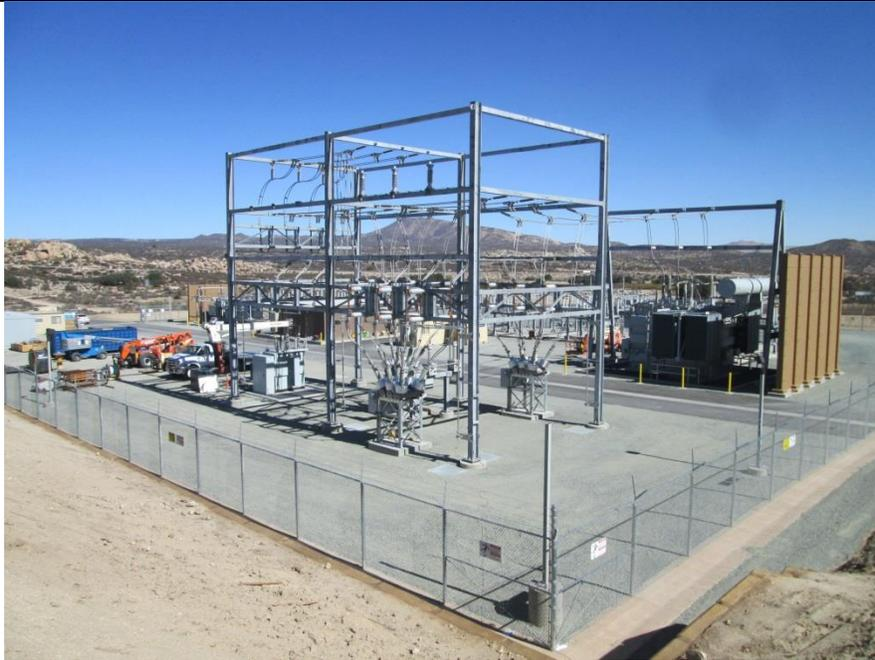
**Photo 5:** A transformer fire wall has been constructed at the Boulevard Substation Rebuild along the southern limits of the substation in accordance with MM-FF-4 and the Fire Protection Plan.
